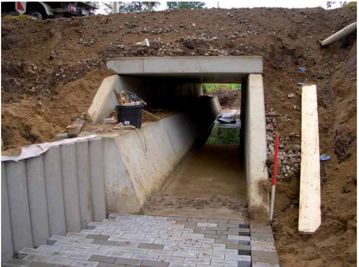
Four concrete precast elements make up the federal road crossing for otters and the Moorsaalweide brook with a total length of 17.4 metres and a width of 2.4 metres.
