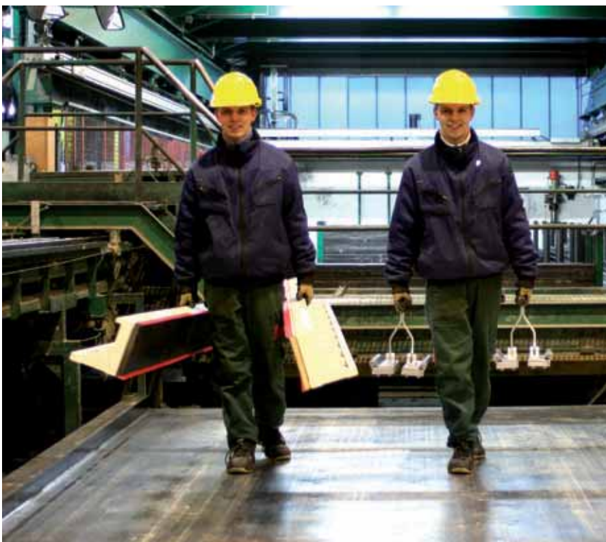
2 employees with 6 m formwork (FlyFrame and formwork shell) and 4 magnets (MagFlyAP)
