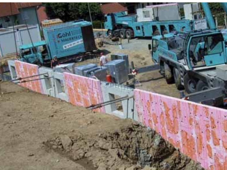
Göhl-Bau installs the exterior basement walls
